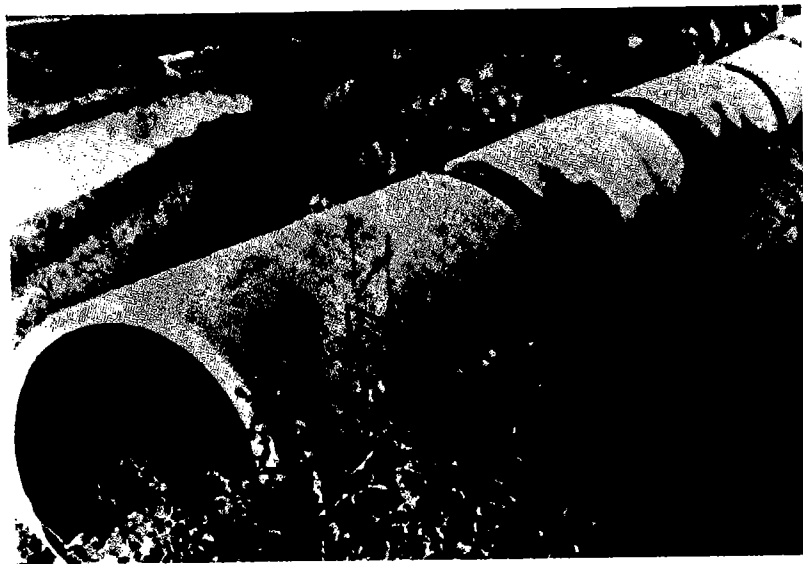
Fig. 15--Waste water piping of self-supporting resin concrete pipe cores
