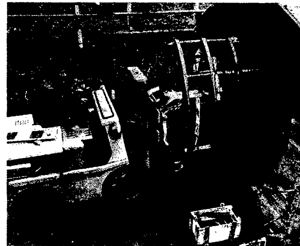
Fig. 28--Mounting of the cages on adjustment bolts and fastening of vibrators
