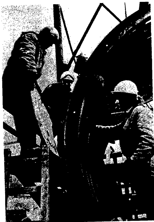
Fig. 22--Placing of resin concrete segments on steel shuttering cages
